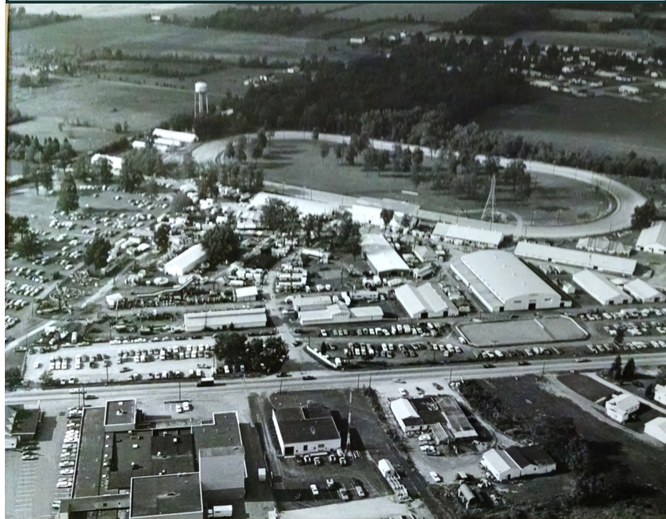
Aerial view of Fairground—1970
